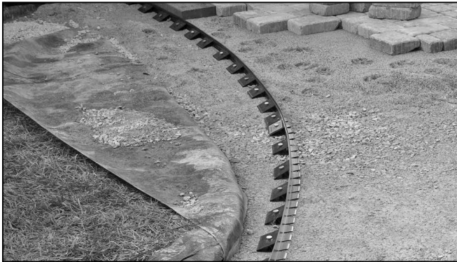
Install edge restraints.
