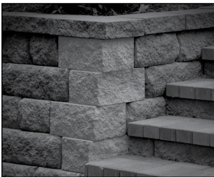
Outside 90-Degree Corner with Corner/Column Unit
