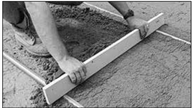
Install bedding sand.
