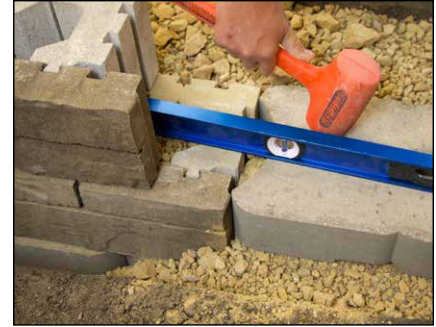
Diagram 7—Stepping up the base
