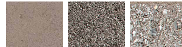
Smooth Shot Blast Ground Face
