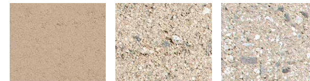
Smooth Shot Blast Ground Face
