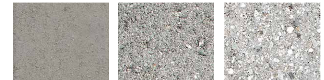
Smooth Shot Blast Ground Face
