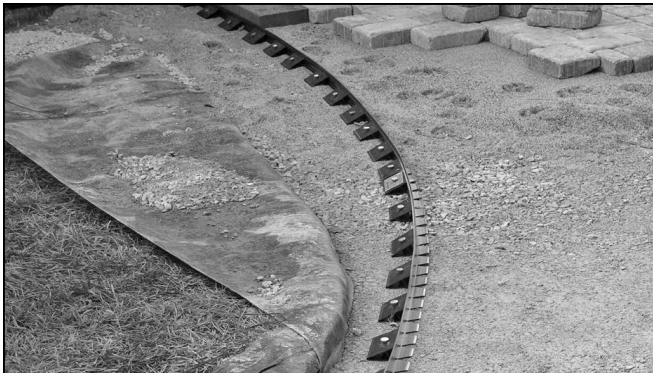
Install edge restraints.
