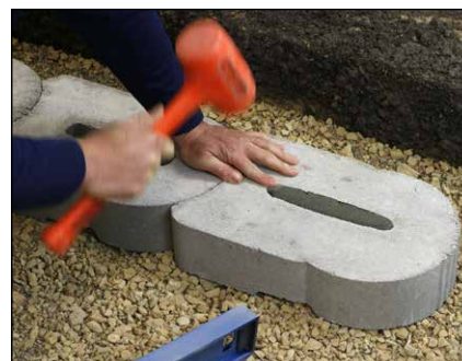
Diagram 3—Lay and level base block
