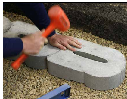
Diagram 19—Lay and level base block
