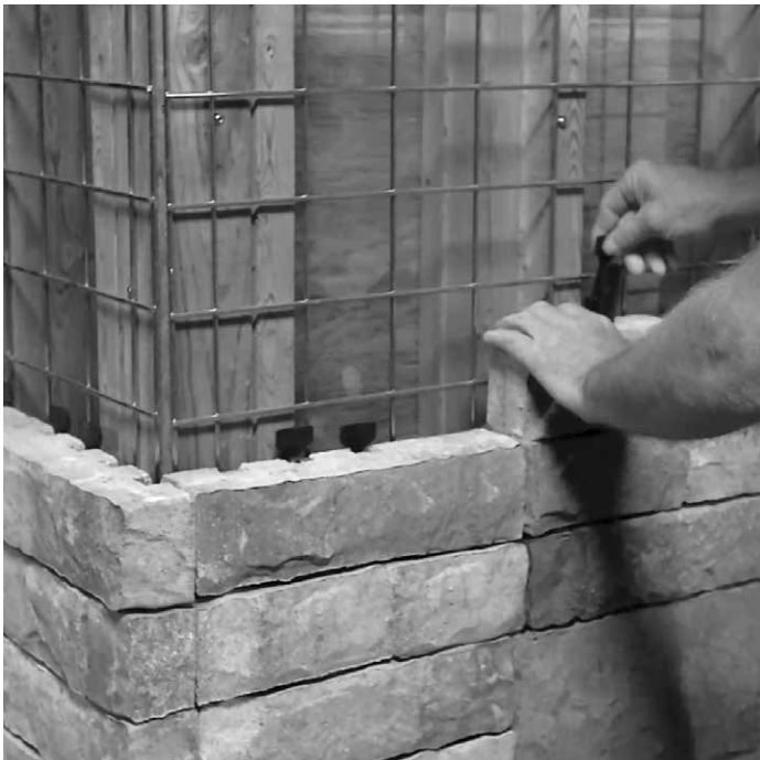
Attach Lafitt Tandem Veneer with Connector
