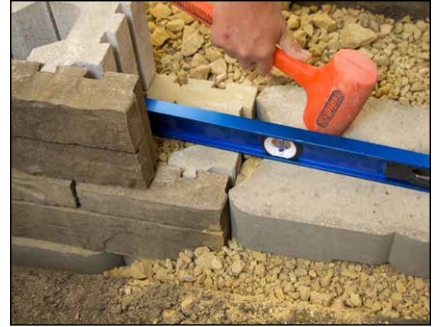
Diagram 7—Stepping up the base
