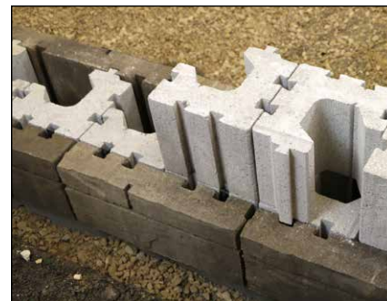
Diagram 21—Second course construction
