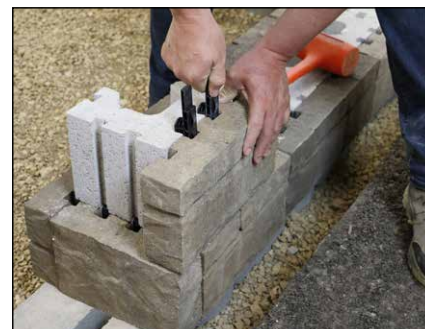
Diagram 22—Wall end example
