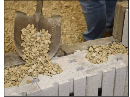
Diagram 5—Fill cores with free draining aggregate
