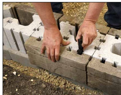
Diagram 20—Placing veneers onto modular block
