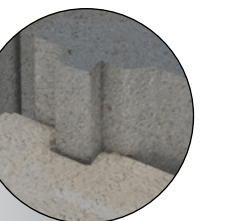
Tenon and mortise on one side
