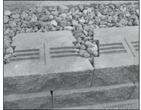
Diagram 6 - Backfill and Fill Voids
