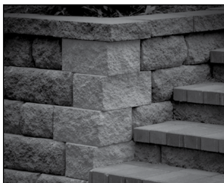
Outside 90-Degree Corner with Corner/Column Unit
