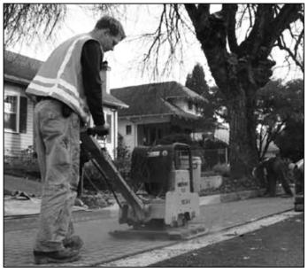
PICP paver compaction shows that pavers need to be set about ¾-inch (19 mm) above their final elevation before compaction and ¾-inch (10 mm) after compaction to account for downward movement.
