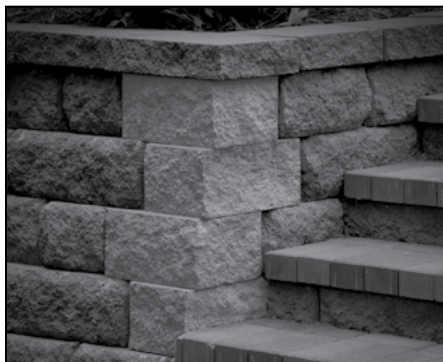
Outside 90-Degree Corner with Corner/Column Unit
