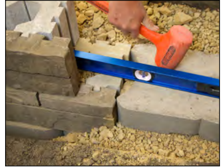
Diagram 7—Stepping up the base
