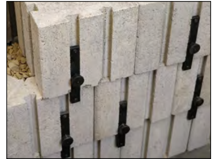
Diagram 6—Lock connector to the block in front
