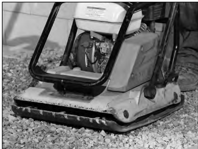
Use 13,500 lbf (60 kN) plate compactor minimum two passes.
