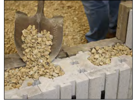
Diagram 5—Fill cores with free draining aggregate
