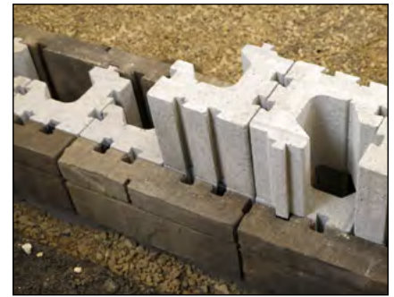
Diagram 21—Second course construction
