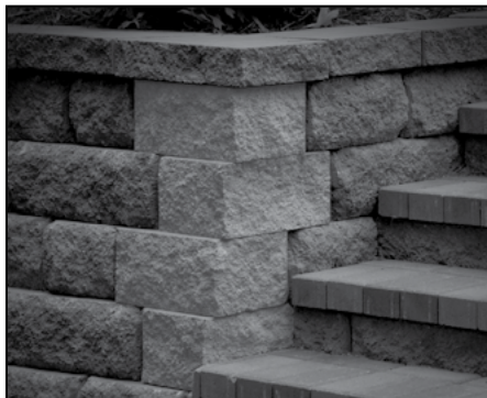
Outside 90-Degree Corner with Corner/Column Unit
