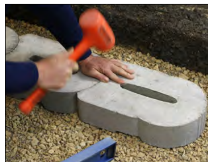
Diagram 3—Lay and level base block
