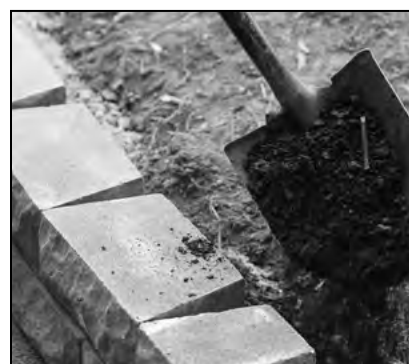
Diagram 2 - Backfill and Compact
