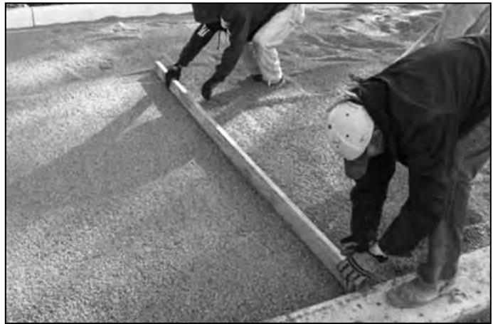
Manually screeding the No. 8 stone setting bed.
