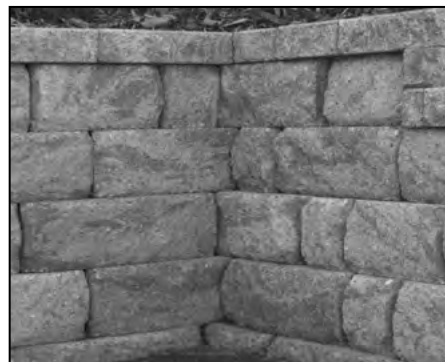
Example Inside 90-Degree Corner
