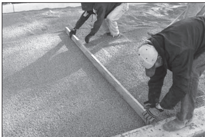
Manually screeding the No. 8 stone setting bed.
