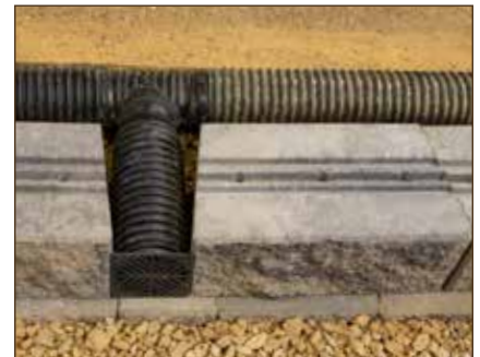
Diagram 7—Drain Pipe Placement
