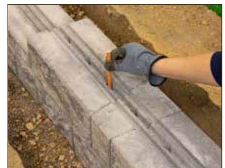
Diagram 16—Pin Placement
