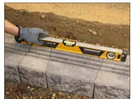
Diagram 4—level each unit
