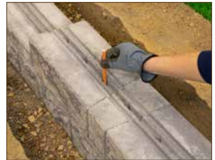
Diagram 6—Pin Placement (Vertical Channel)
