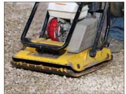
Diagram 14—Leveling Pad
