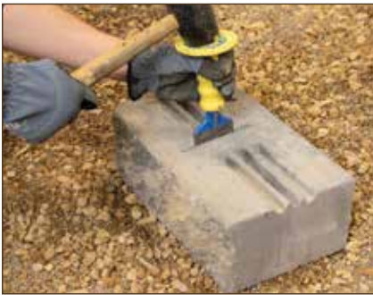
Diagram 17—Split block in half
