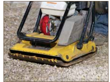
Diagram 2—Leveling Pad
