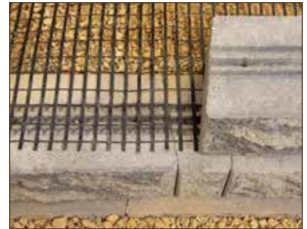
Diagram 9—Reinforcement
