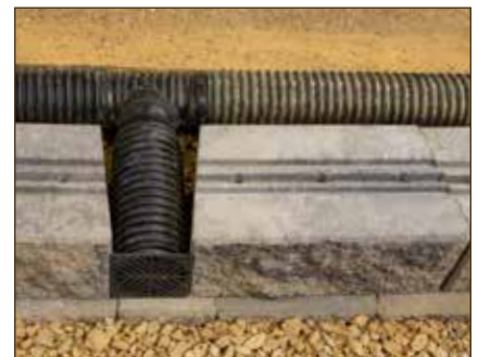
Diagram 7—Drain Pipe Placement*
