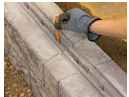
Diagram 6—Pin Placement (Vertical Channel)*
