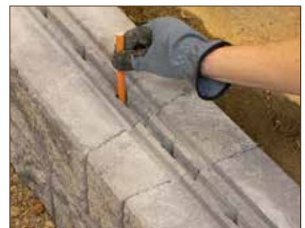
Diagram 16—Pin Placement*
