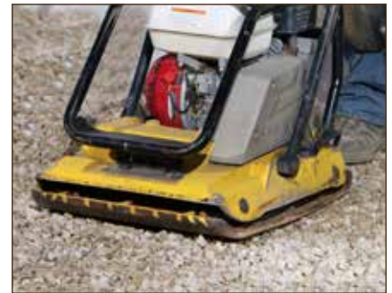
Diagram 14—Leveling Pad
